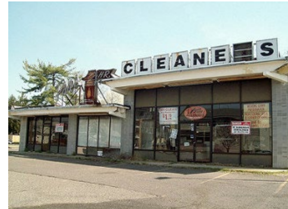
Former Dry Cleaners
