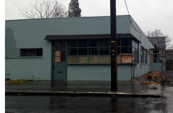
Vacant Commercial Building
